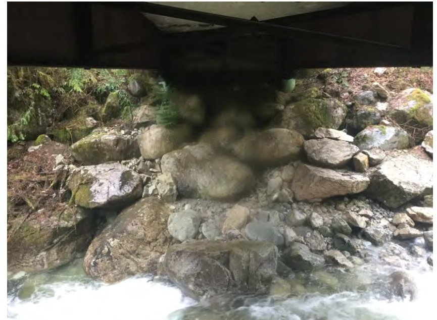
Right Bank Abutment when facing downstream
