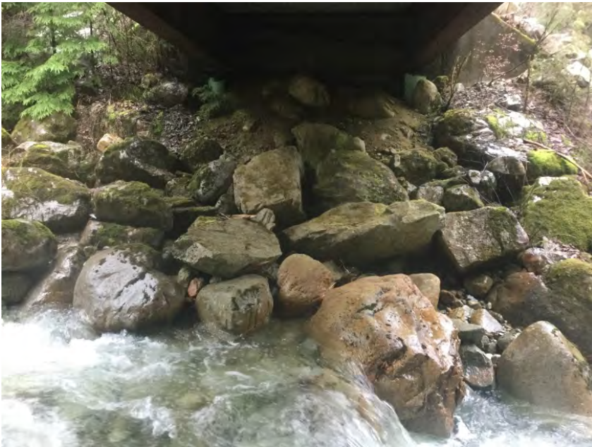
Left Bank Abutment when facing downstream
