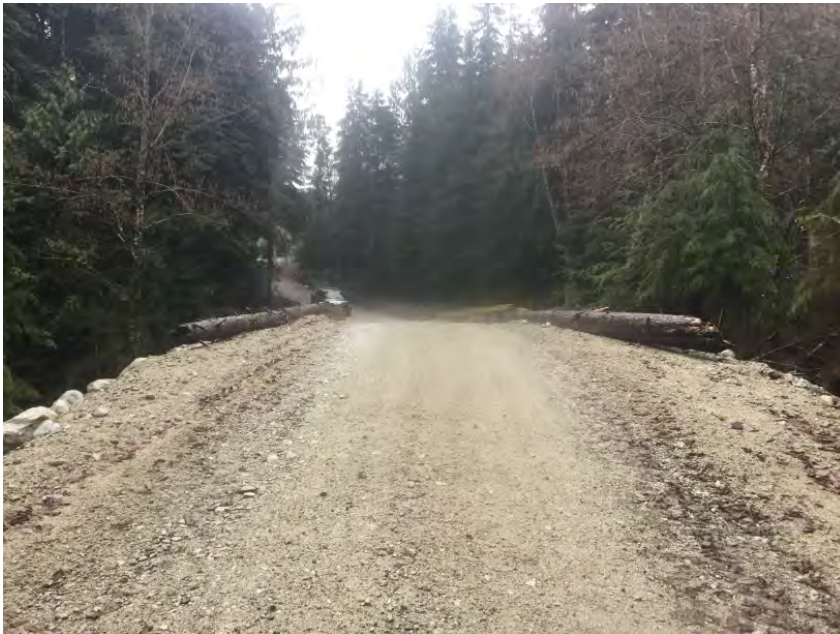
Approach from Left Bank when facing downstream
